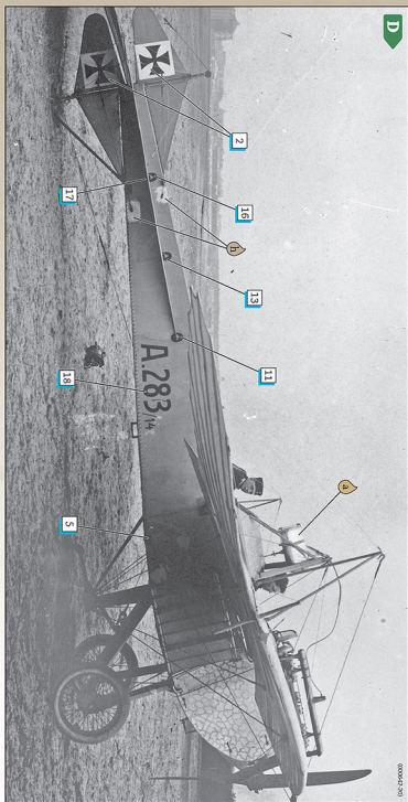
Jeanette Stahlbau 283/14 photographed at Adlerhof-Johannisthal. Note the recent alterations or repairs to the rudder control cable exits in the rear of the fuelage. If these patches are CDL, then it is strong evidence for the rest of the fuelage being finished in field grey.
