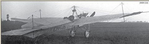
85hp Daimler-Mercedes D6f (precursor of the 100hp D.1) powered Etrich Taube "D2" in 1913.
